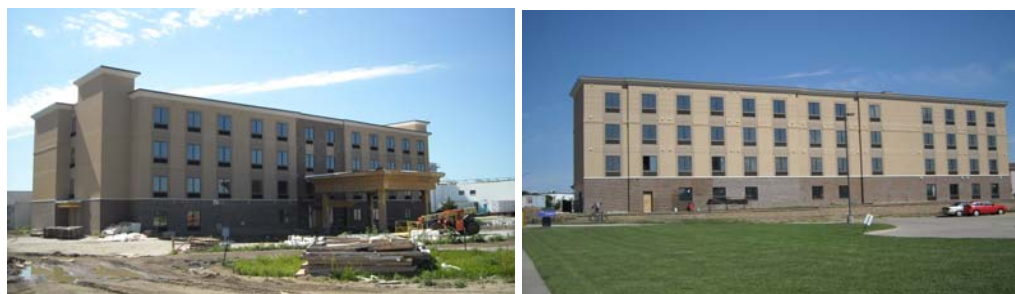
Holiday Inn Express, Under Construction, Lincoln, Nebraska, 2007
